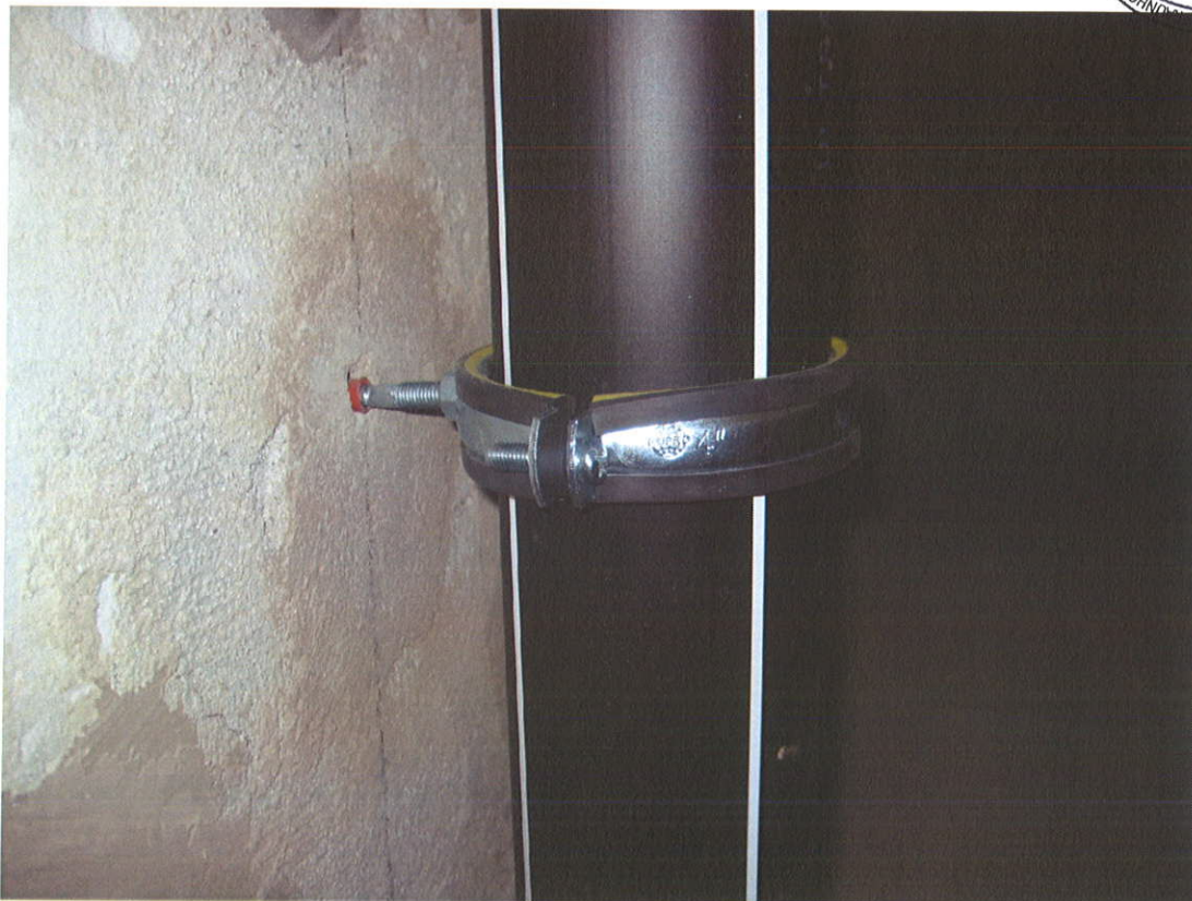
Figure 5 Waste water system "Ultra Silent+ 110 x 4.8" with pipe clamps "Müpro yellow, with spacer 5 mm".
